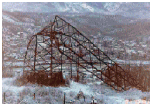
Figure 1 - Damage of towers of power lines
